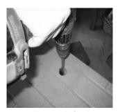
Drilling a Hole for the Gas Line
