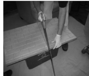
Cutting the Panel to Size
